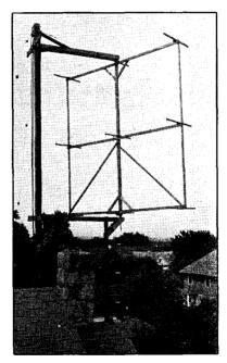
FIG. 1633—THE 112-MC. ARRAY AT W2CUZ: AN EXCELLENT EXAMPLE OF CONSTRUCTION TO ALLOW ROTATION OF THE SYSTEM
