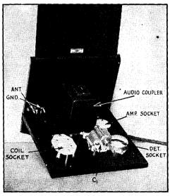
FIG. 706 - TOP VIEW OF THE BASE ASSEMBLY
